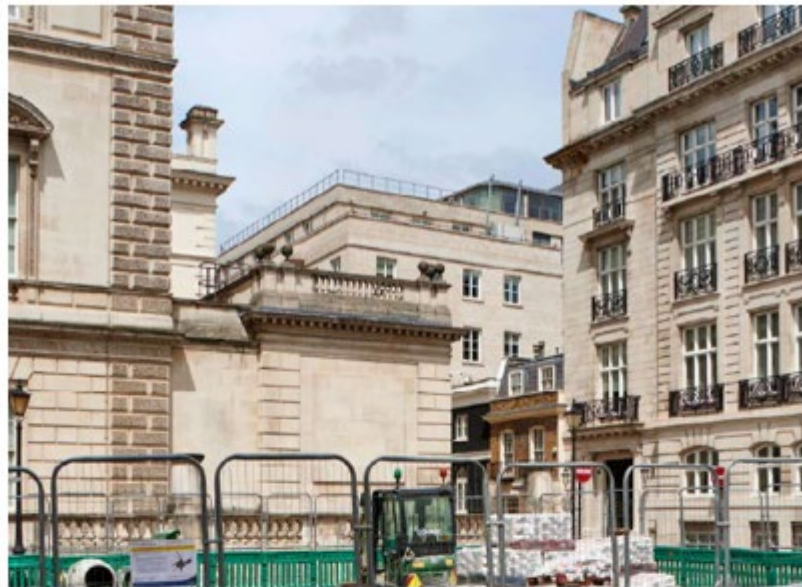
Existing view (above) from Cleveland Row
